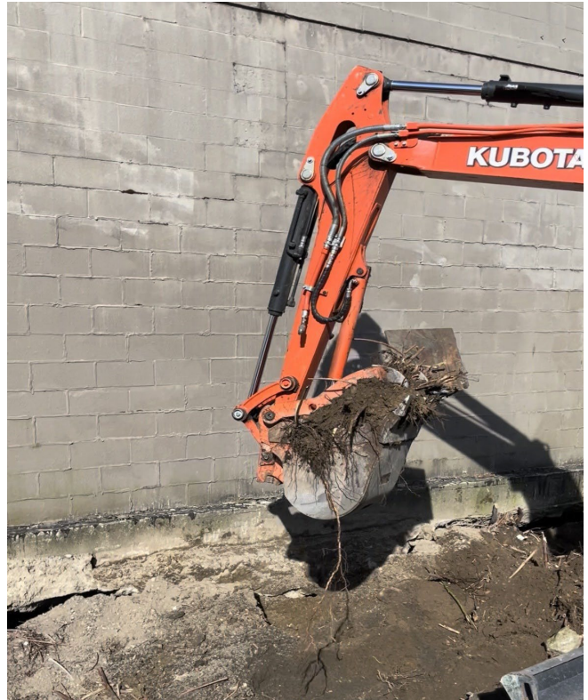
Excavation and treatment under controlled conditions
