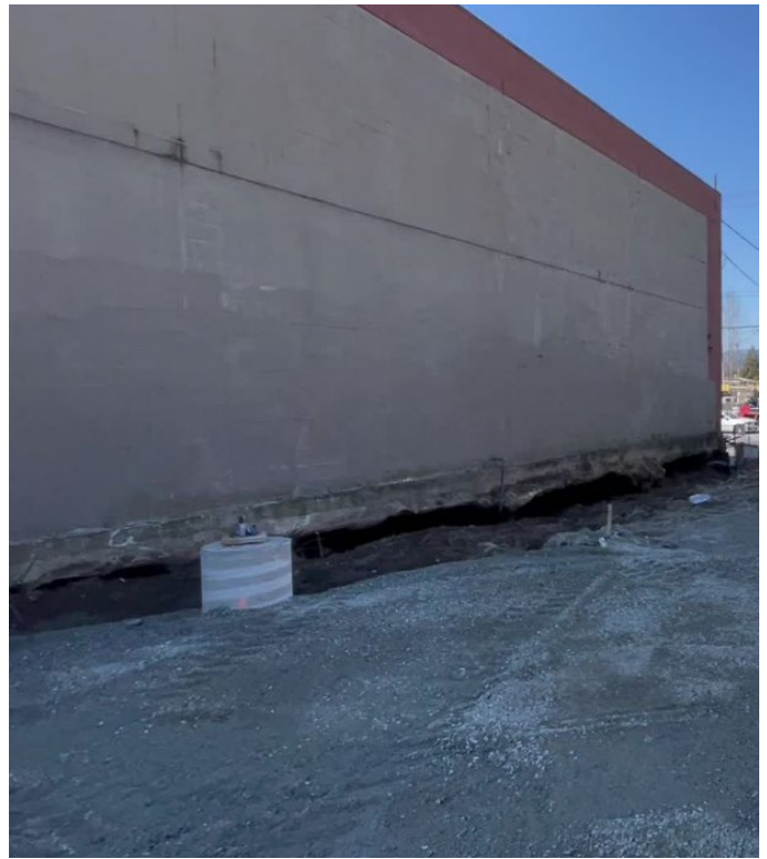
Site clean and free of Japanese Knotweed
