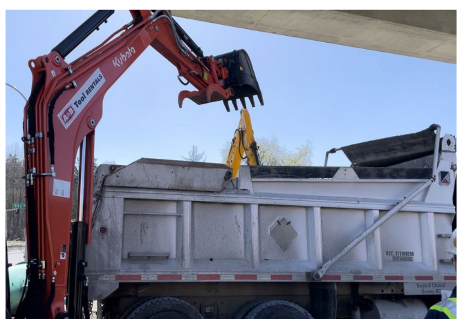
Disposal via dump truck to a suitably licenced facility
